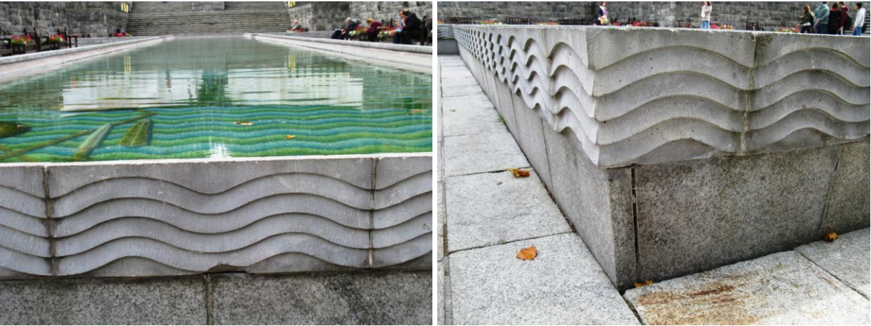
View of granite and limestone boundary to pond.
